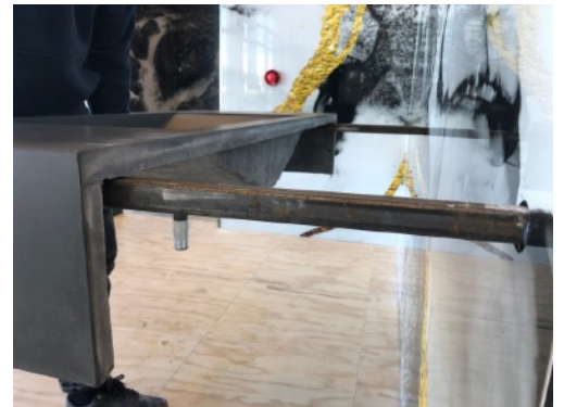
Deposit the vanity on the bracket
