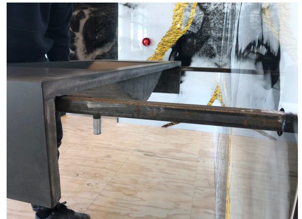
Deposit the vanity on the bracket
